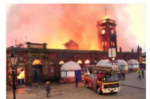
Ashton-under-Lyne market hall is damaged by fire.
