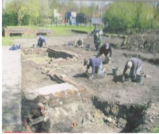
The foundations of the new single-storey range added to the barn.
