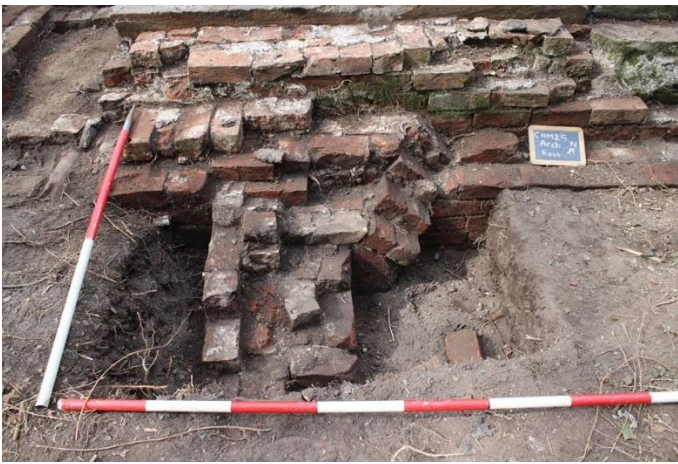
Plate 11: Truncated wall and springer for brick arch in Test Pit 3 on eastern side of engine bed. Plate 12: Brick wall and stone pads on east side of engine bed.
