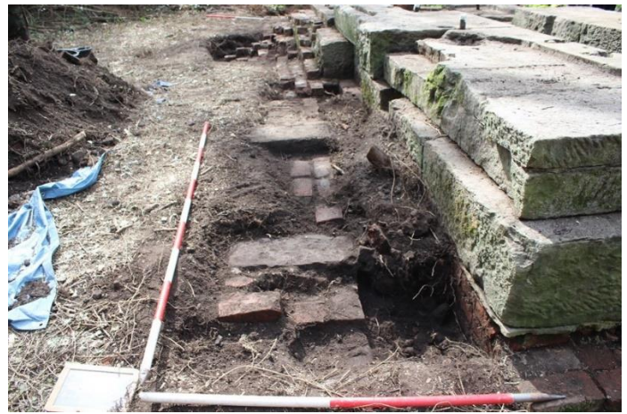
Plate 11: Truncated wall and springer for brick arch in Test Pit 3 on eastern side of engine bed. Plate 12: Brick wall and stone pads on east side of engine bed.
