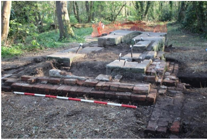
Plate 9: Southern end of engine bed showing wall projecting to the south. Plate 10 (right): North east corner of engine bed, showing reuse of corn drying kiln tiles in the lower level of grey tiles at the foot of the brick work.
