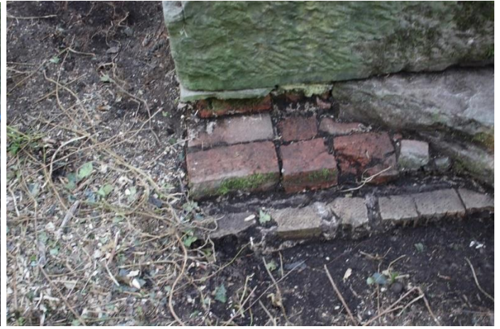
Plate 9: Southern end of engine bed showing wall projecting to the south. Plate 10 (right): North east corner of engine bed, showing reuse of corn drying kiln tiles in the lower level of grey tiles at the foot of the brick work.
