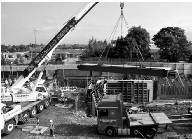
Crane lifting the Footbridge into position – photograph courtesy of GMPTE
