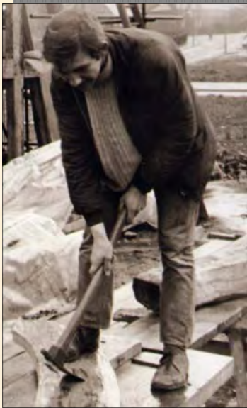
An adze being used on the new oak cruck truss
