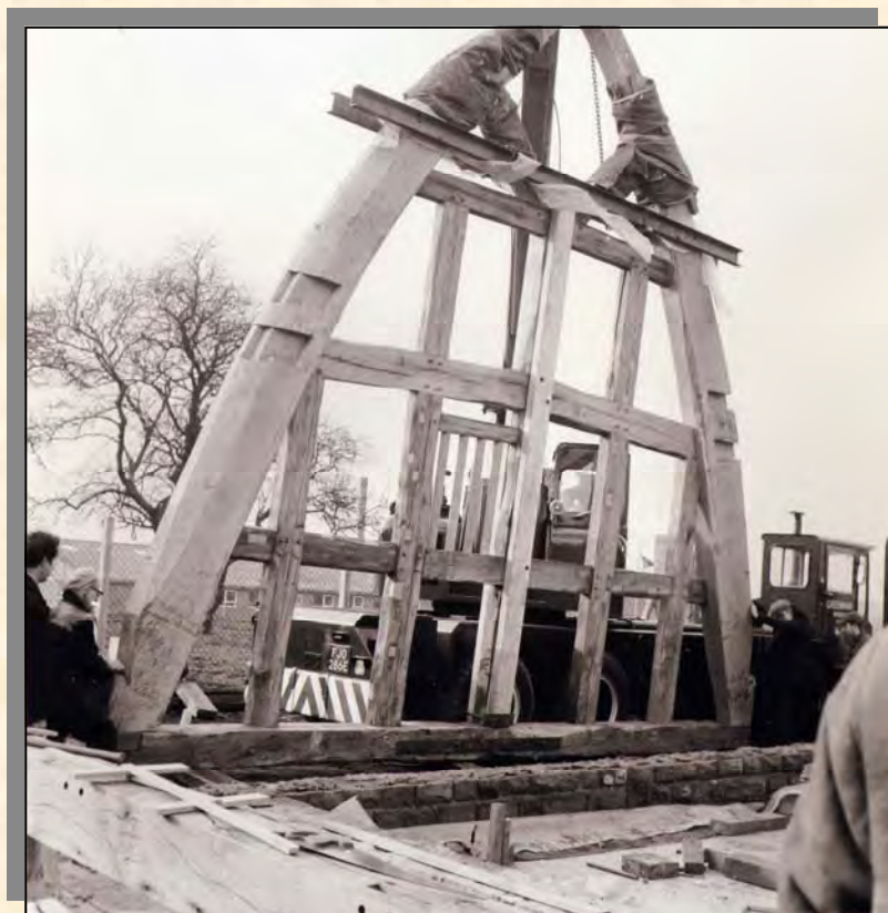
Erecting the new oak cruck truss in 1968
